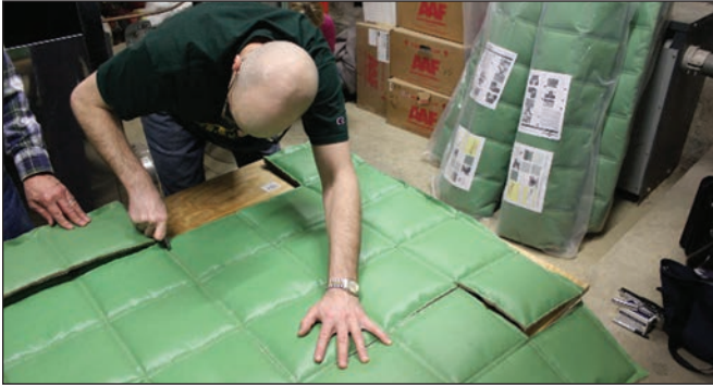
Photo 4: A worker cuts pieces from a 4 ft x 8 ft (1.2 m x 2.4 m) sheet from a modular insulation kit. Once cut to size, the insulators will use strips of hook and loop fastener tape, stapled to the pieces, to secure them around the component being insulated.
